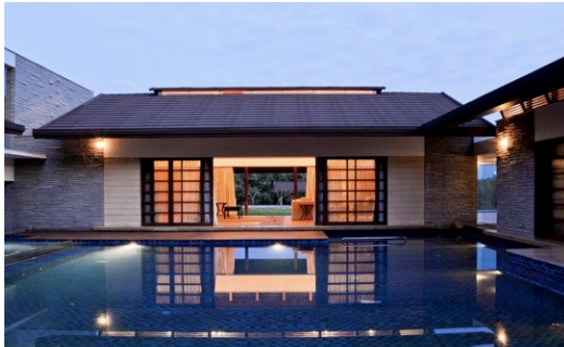
CnT Architects: Ramaiah House, Bangalore, India. A quest for a timeless aura
